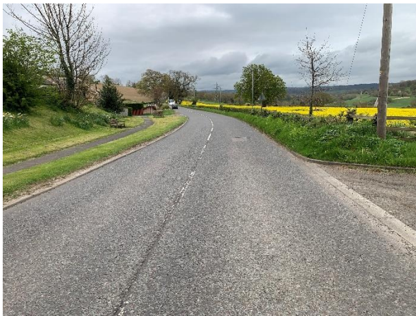
Photo 15 – A6079 view south end of village towards the end of the 30mph speed limit
