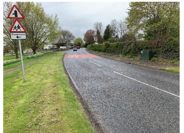
Photo 10 – A6079 north entrance to village showing 30mph speed limit signs and roundel
