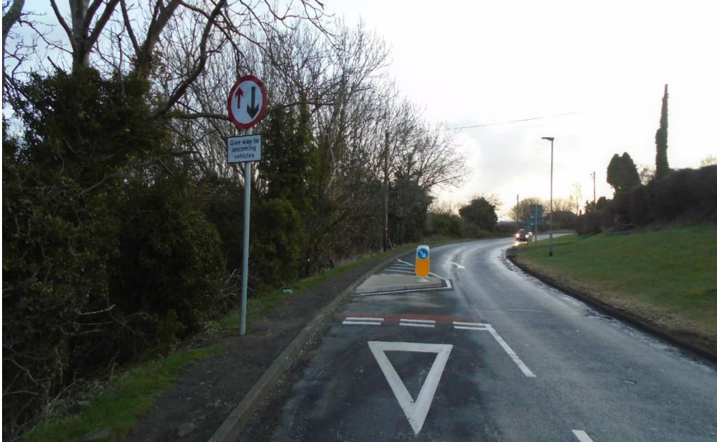
Photo 22 – Example of single build out priority working chicane at New Ridley
