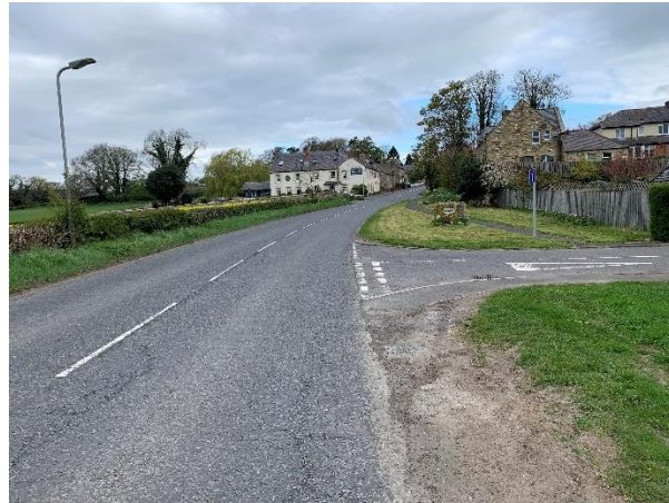
Photo 3 – A6079 south entrance to village showing stone village nameplate sign
