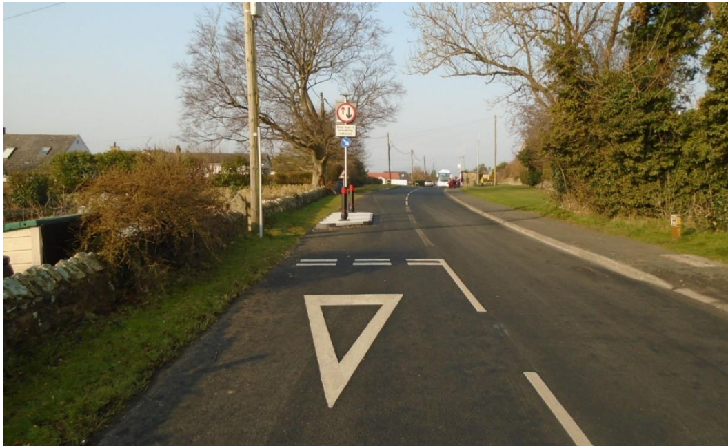
Photo 21 – Example of single build out priority working chicane at Longframlington
