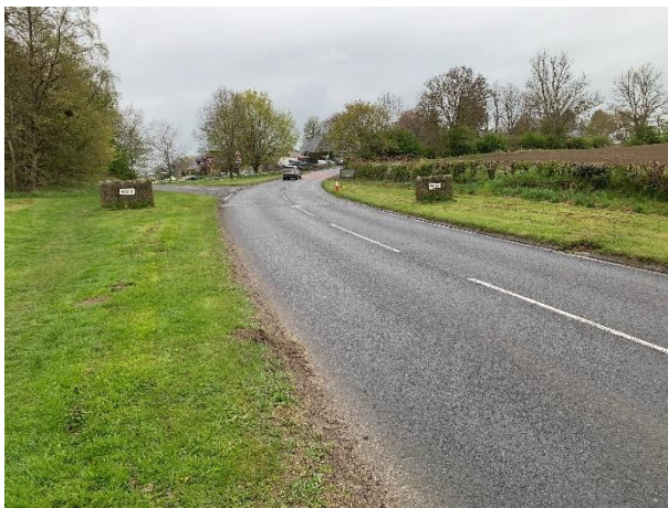
Photo 9 – A6079 north entrance to village showing stone village nameplate signs
