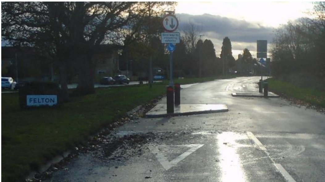
Photo 18 – Example of dual build out priority working chicane at Felton
