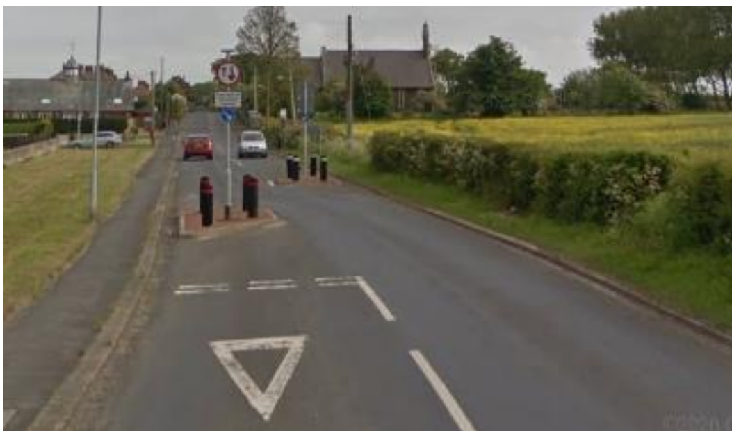
Photo 19 – Example of dual build out priority working chicane at Hadston
