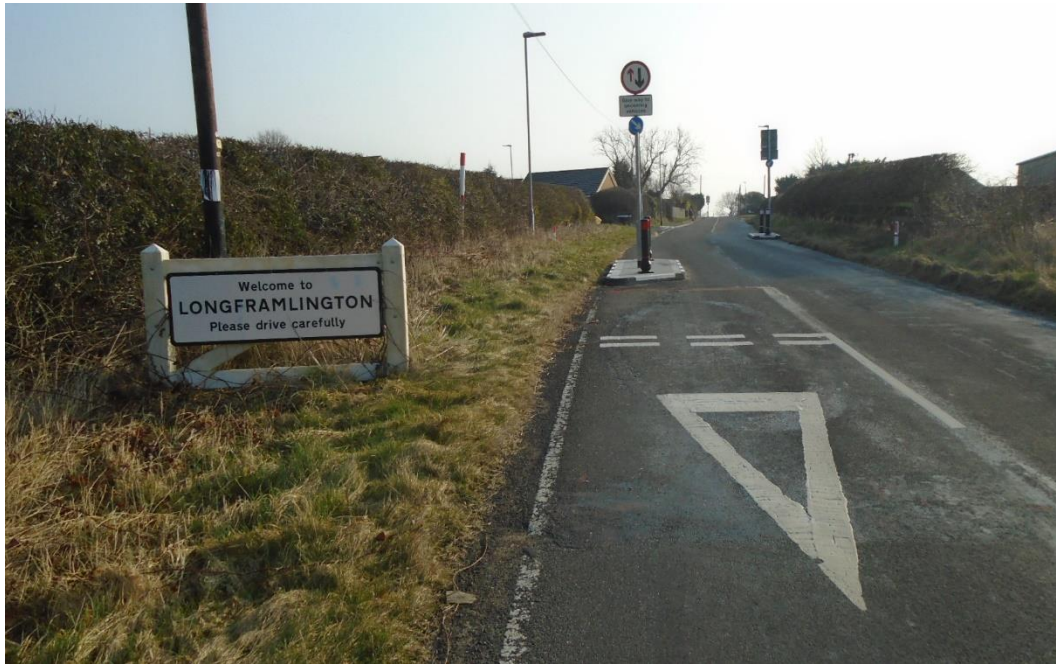
Photo 20 – Example of dual build out priority working chicane at Longframlington
