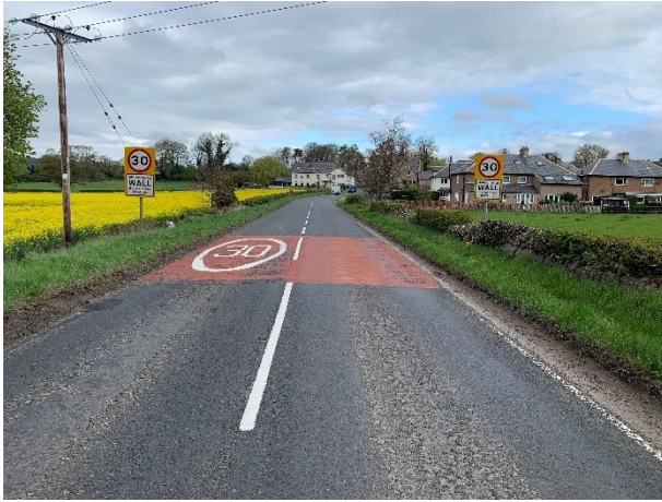
Photo 1 – A6079 south entrance to village showing speed limit signs and roundel
